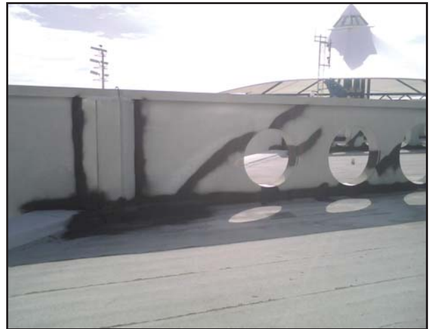
SEALING CRACKS IN CONCRETE WALLS
