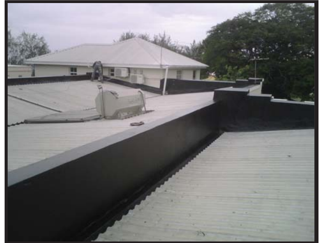
SEALING A PARPET WALL BEFORE TOP COAT APPLICATION
