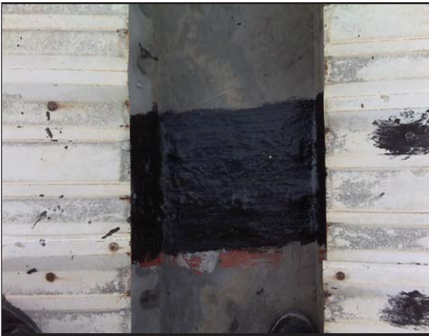
SEALING METAL GUTTER JOINT
