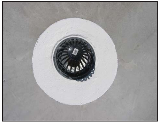
TROWEL GRADE & TOP COAT SEALING A DRAIN IN A CONCRETE ROOF
