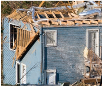
Blown off roof
