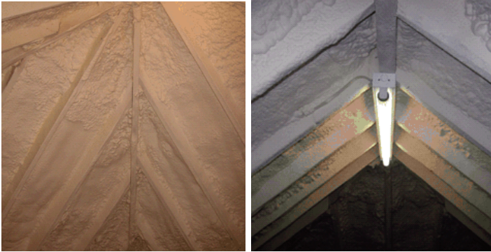
Closed cell SPF applied to the underside of a roof increases the racking strength
