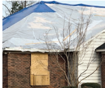
House is still standing, but the roof has been torn off
